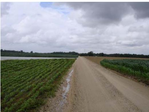
PURE CRETE treated road base, with increased density and cohesion of smaller soil particles, resists the penetration of moisture and eliminates the ability of soil particles to migrate within the road material. The reduction of moisture decreases the plasticity of the material - reducing road deformation under wheel loads.
