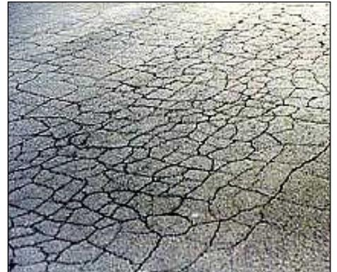
When the clay fines (-200 mesh) exceed 25% or are highly expansive some surface cracking will occur. Generally the cracks are superficial, often filling in with road particles during normal traffic use. Generally this condition is referred to as "Alligator Cracking" and does not significantly affect the stability of the road base.
